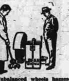
We Also Have This Bean Wheeler Balancer to Check the Balance of Your Wheels. Unbalanced wheels have been known to throw the car out of con-trol to such an extent that it would leave the road or a collision would result.
